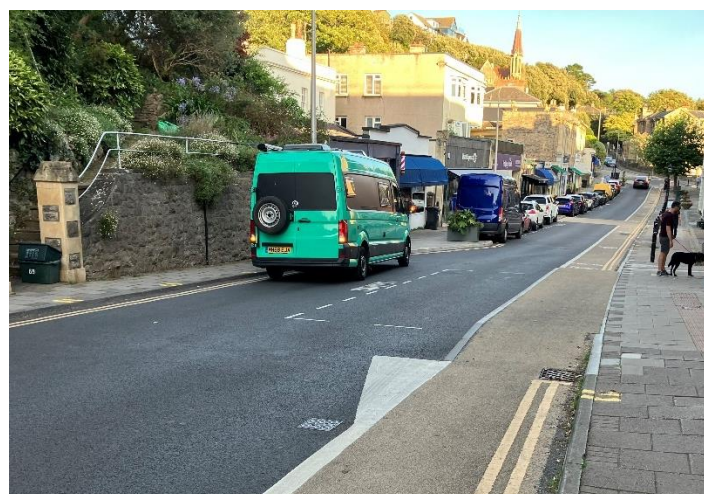
Figure 24 – Vehicle stopping outside loading bay
